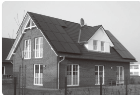
Solar/home power supply
